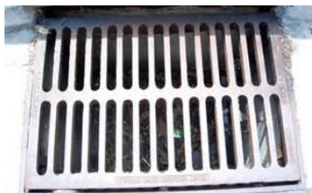
Storm Drain Grate
