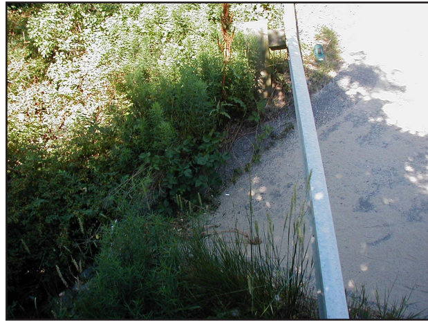
Paved Stormwater Swale on Route 28
