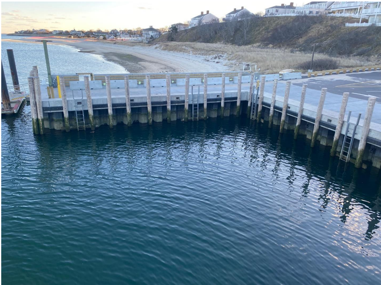
New Bulkhead along South Jog.
