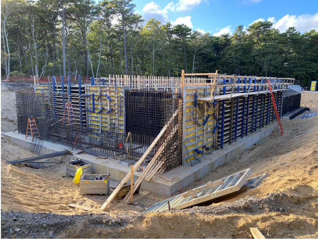
Foundation Walls Formwork at Wells 5 & 8 PFAS Water Treatment Site
