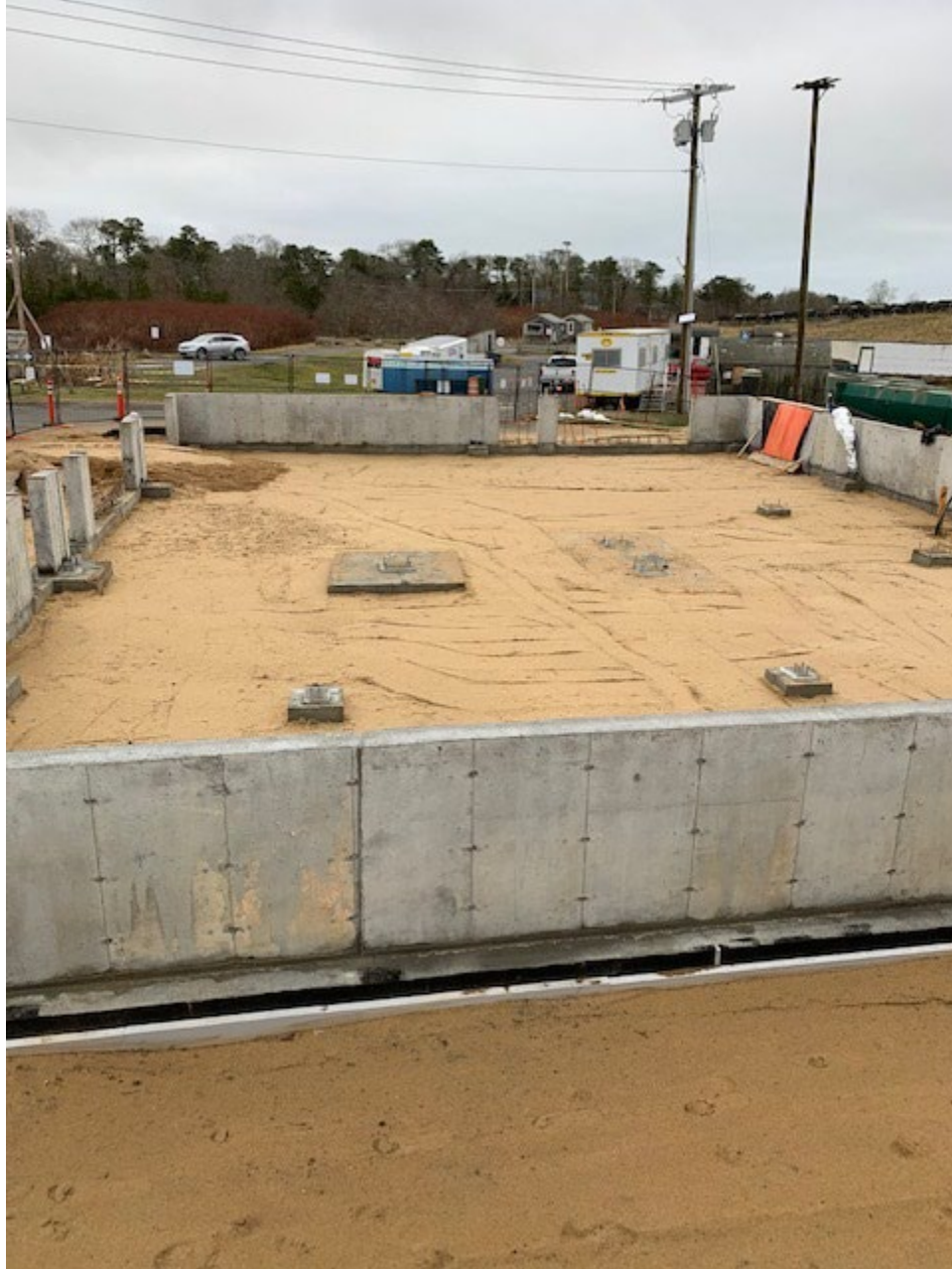
Foundation work at Transfer Station – Phase II (Priority I)
