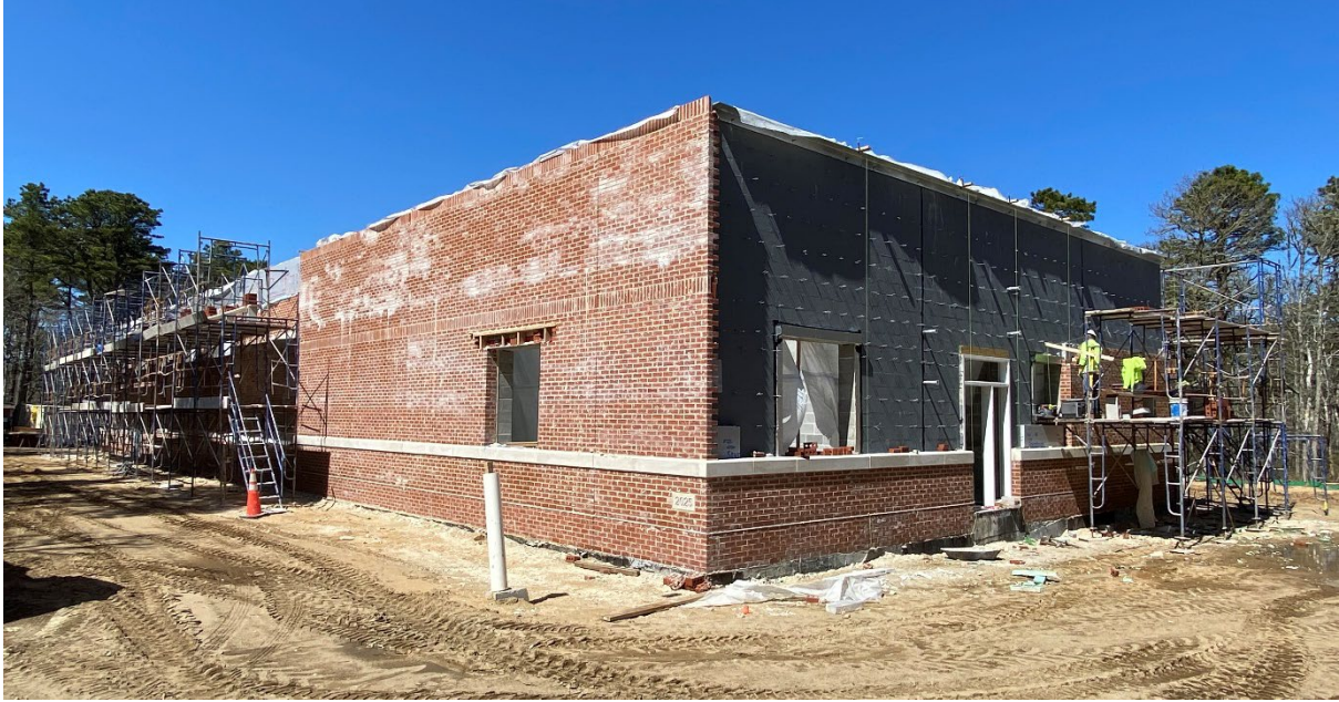
Wells 5 & 8 Treatment Plant – Exterior Brick Work
