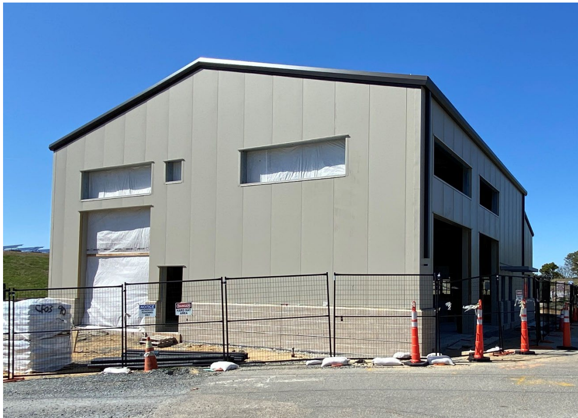
Building Envelope Construction at Transfer Station – Phase II (Priority I)
