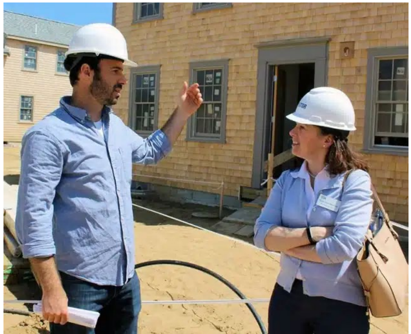
VP of Real Estate Development, David Quinn, on construction site at Sagem's Path Nantucket (Completed in 2018)
