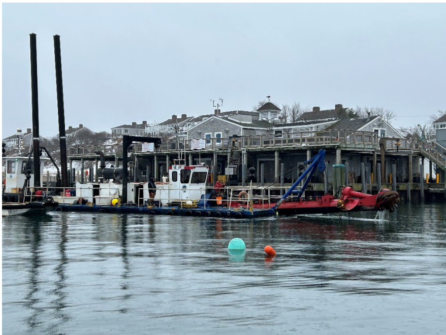
Left: Barnstable County Dredge "Sand Shifter" at Aunt Lydia's Cove
