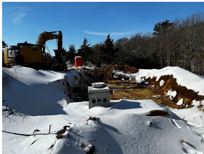
(A snowy overdig site. The upper soil horizons were excavated and removed, making way for the installation of a Title 5 soil absorption system.)
