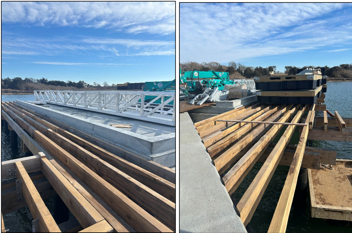
Above: Stringers placed for Decking around Boathouse (01/22/26)
