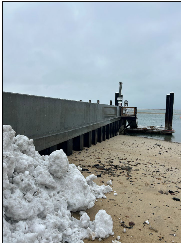
South Jog Walkway Pre-Construction 2/25/26
