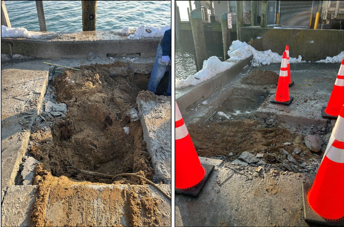
North Jog Cut Landward Side of Bulkhead (2-11-26)
